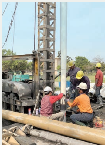
鑿井工程 Well drilling engineering
