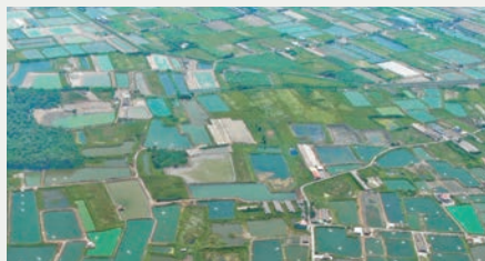
養殖輸水工程 Water Supply engineering
